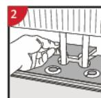
Drill holes two times larger than the diameter of the pipes. Remove a piece of the panel with a utility knife. Put the panel on one side of the pipes and the removed piece on the other side.
