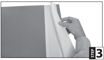
**Step 3:** Be sure to unfold the film, extending it 3" from the foam.
